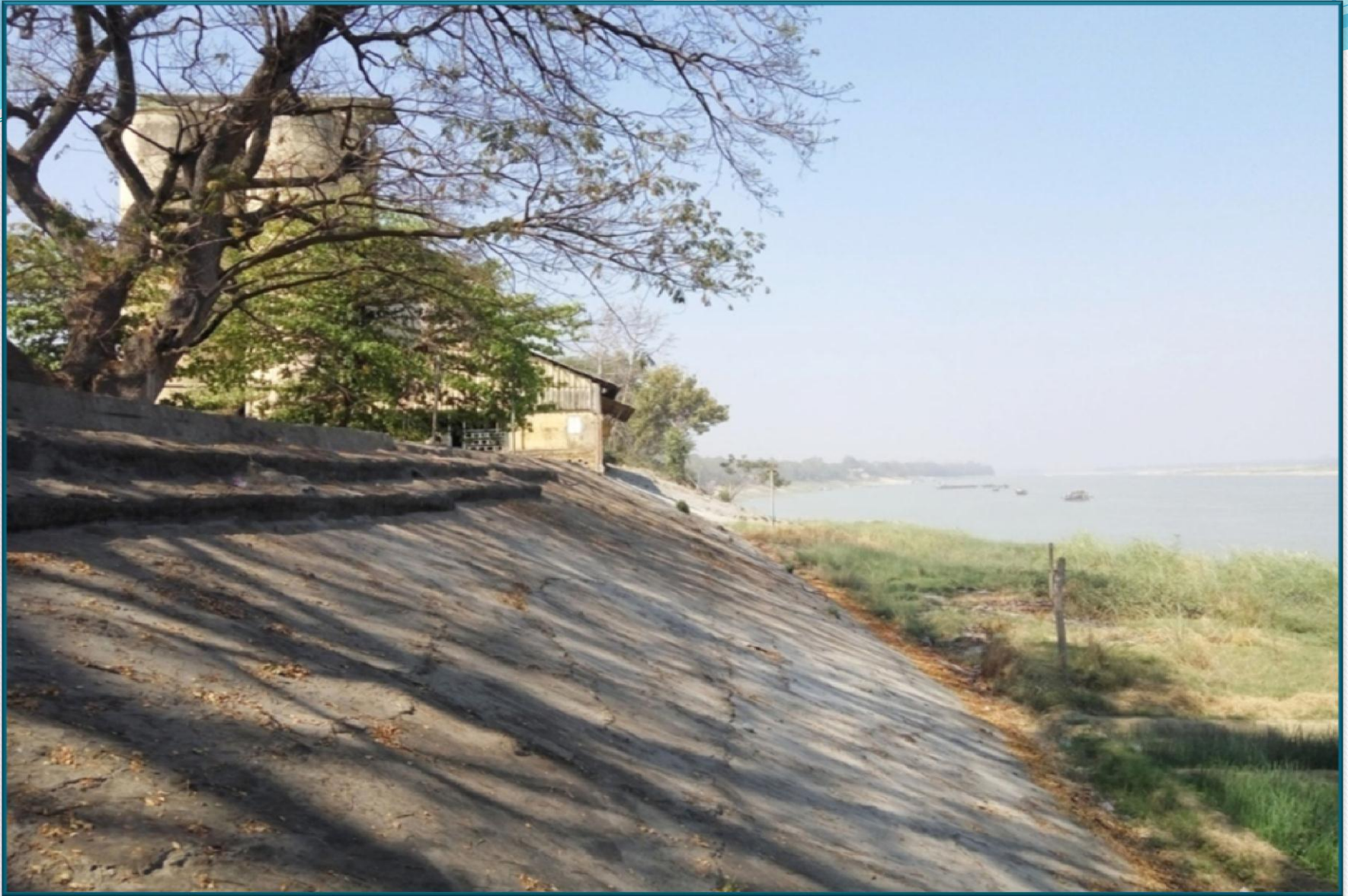
No.(31) Heavy Industry (Thayet) Concrete Embankment for Flood Protection
