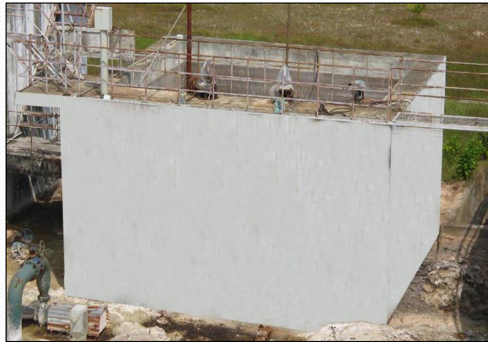
Primary Sludge Tank ( 6m x 6 m , Depth -5m )
