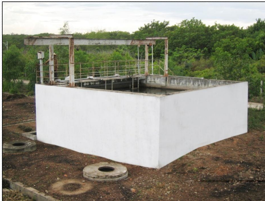
Secondary Sludge Tank ( 8 m x 8m , Depth -5m )
