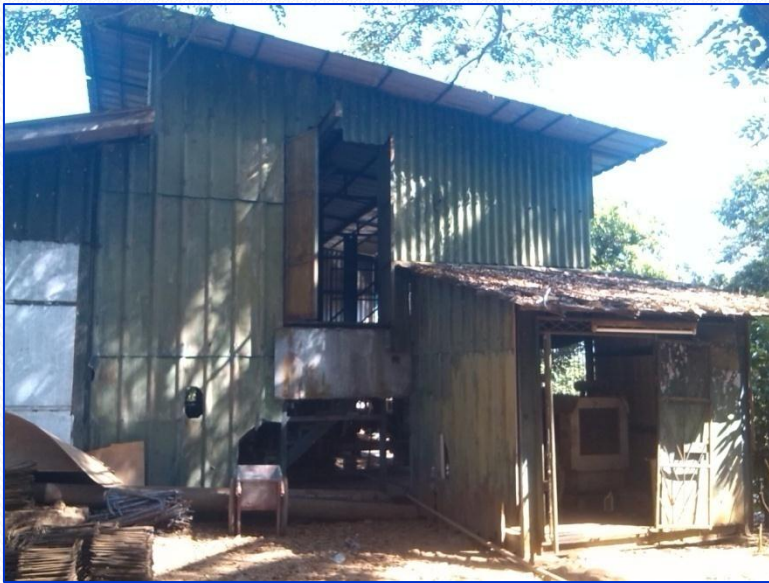
Raw Water Pumping Station
