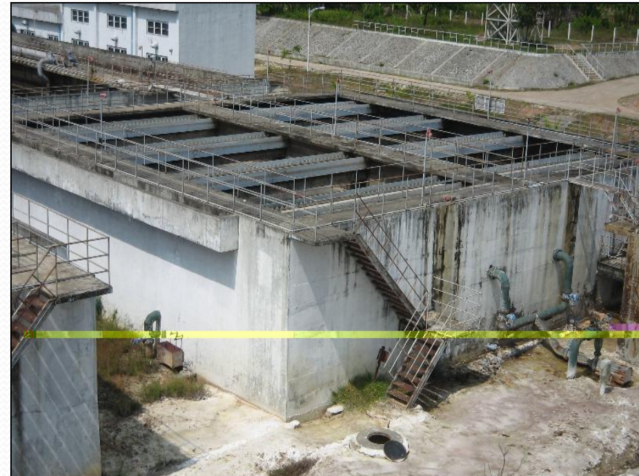
Hydrolysis Tank ( 25m x 17 m, Depth 6m x 2 Nos)
