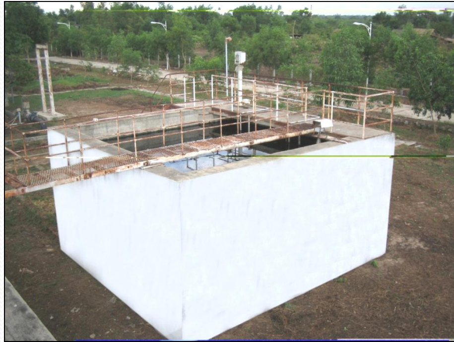
Excessive Sludge Tank ( 5 m x 5m, Depth -4.5m )
