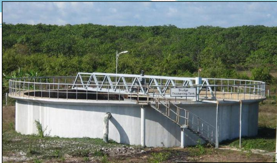
Sludge Thickener ( \phi 17m , Depth -3m )
