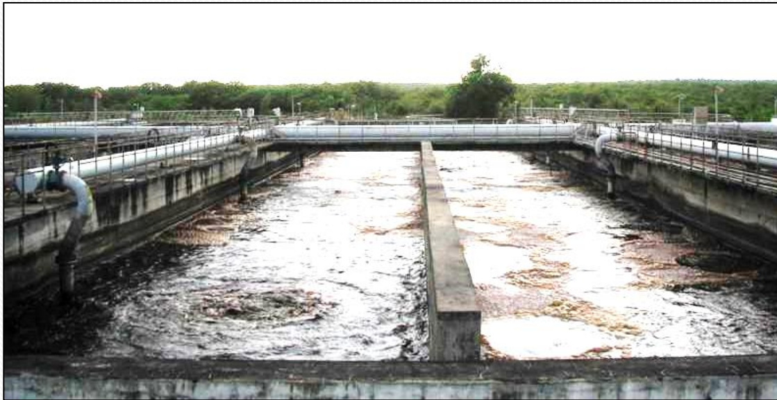
Aeration Tank ( 73.5 m x 24 m , Depth -9m - 2 Nos )
